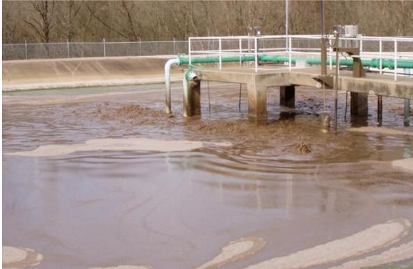
**Jet Aerated Aerobic Digester**
