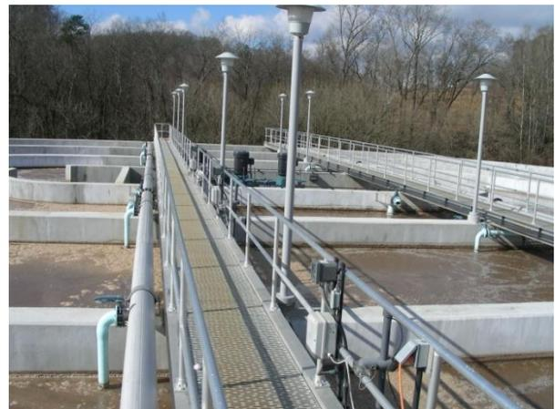
**Air Delivery Piping – Note Butterfly Valve and DO Sensor in Each Channel**
