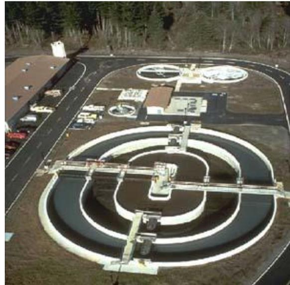
**Multi Channel Reactor with Surface Aerators.**
