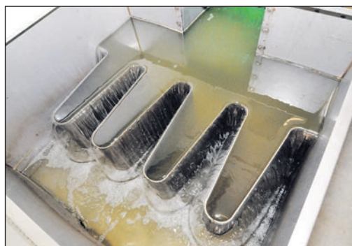
Water is treated by ultraviolet light, the final part of the process which started with raw sewage, which is converted to clean water and safely released back into the ecosystem.
